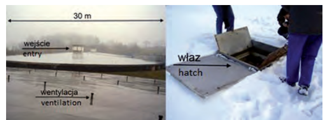
Fig. 2. Tanks for storing water – MPWiK Cracow
